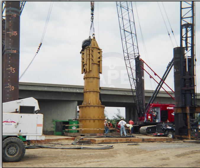
THE APE 7.5A WITH A DIRECT DRIVE BOOT.
