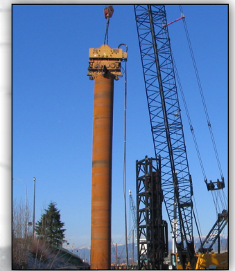
MODEL 600 VIBRO WITH THE D180-42. FINISHING 1.8 M PILES.
