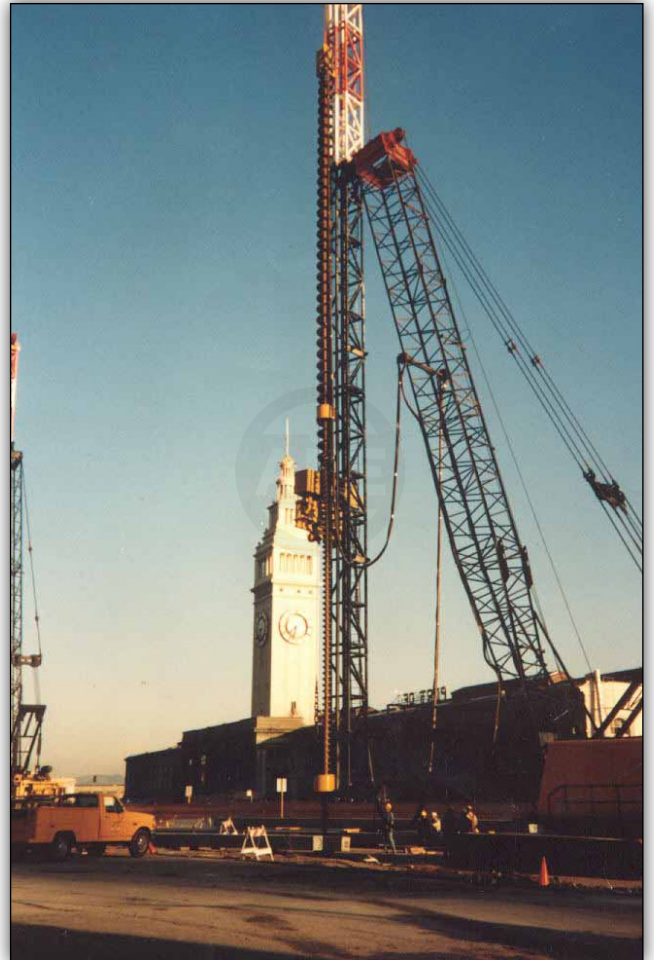
AN APE 75 DRILL IN A PRE-DRILL FORMAT ON THE SIDE OF A FIXED LEADER WITH A KING KONG IN SAN FRANCISCO, CA OWNED BY KIEWIT.
