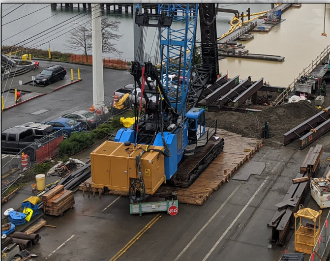
CUSTOM BUILT MODEL 580 POWER UNIT TIER IV RUNNING A 375K DRILL AT SEATTLE, WA FOR ORION.
