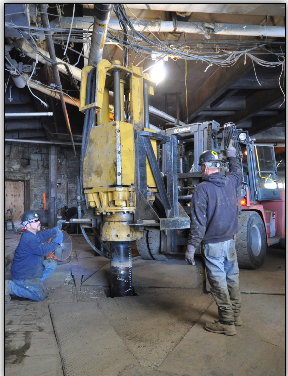
FORKLIFT MOUNTED 7.5 HYDRAULIC IMPACT HAMMER.
