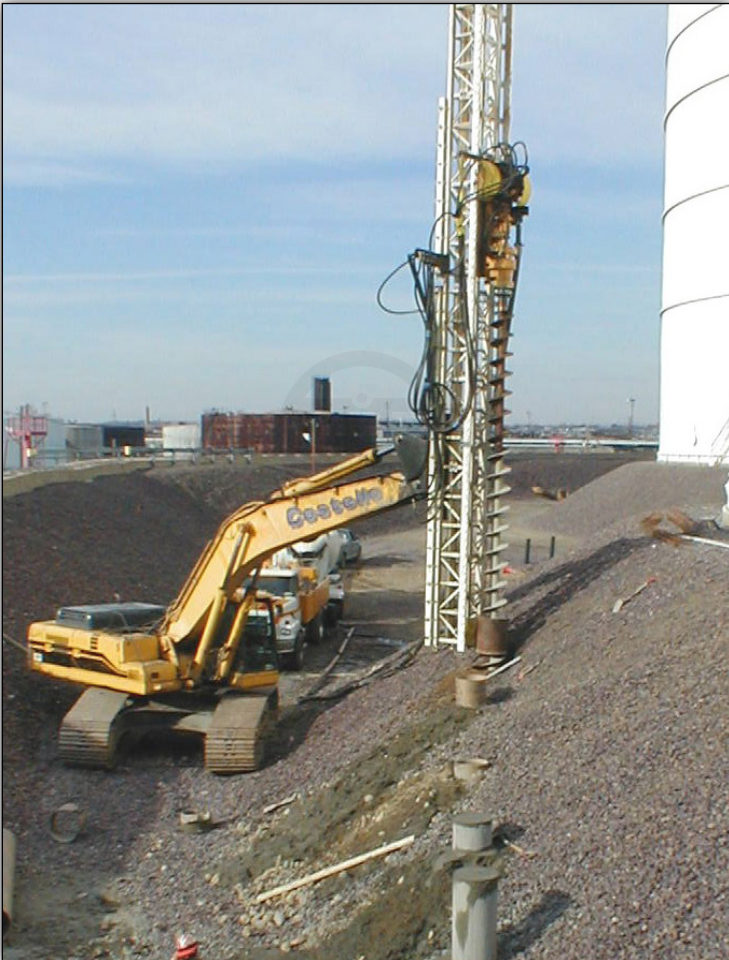
MODEL 20 DRILL MOUNTED ON THE APE RACK AND PINION LEADER WITH 15,000 POUNDS OF CROWD CAPACITY.
