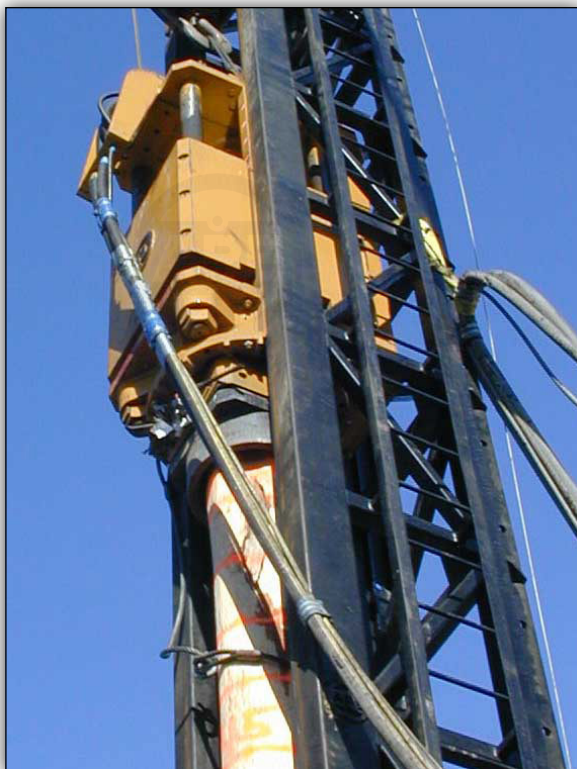
ROUND CONCRETE INSERT FOR CONCRETE PILES.
